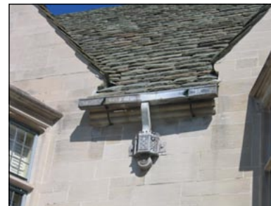
Lead gutters and drain.
