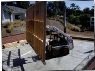
And the next day we had built the first wall (which weighed a ton) so relied on our Bobcat to grab, lift and set the framing on the 6' block wall.
