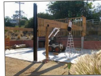
Second beam (a 30 footer) being installed now.
