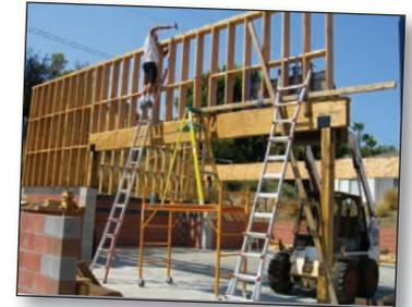
And the next section of the cripple wall. Wall had to be lifted 10'-4" to fit over beam so Bobcat helps again.
