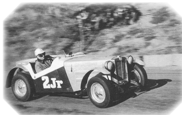
'47 MG TC with Ford V8 60 flathead engine (2.2 liter)
