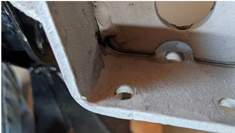
The above bolt hole, repaired.
