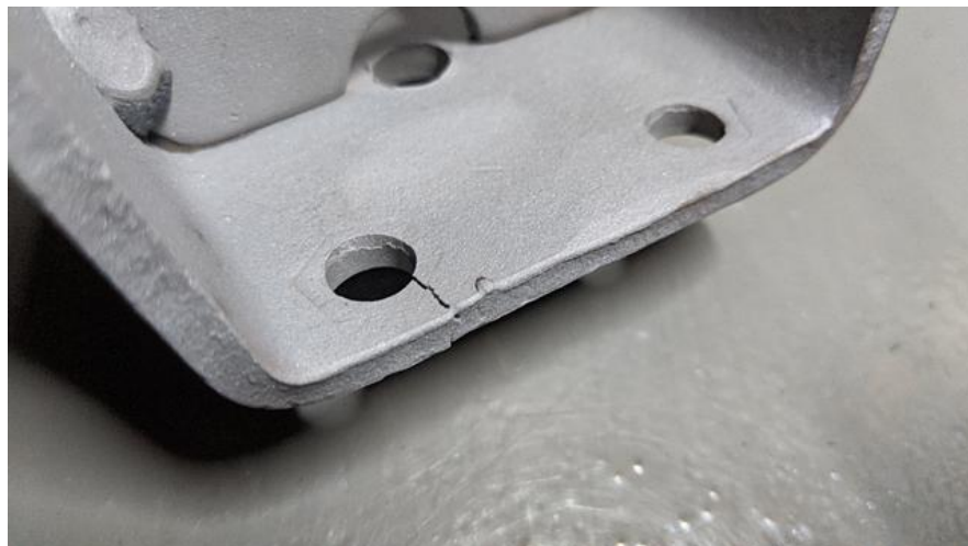
Cracked tower bolt hole. Note how the metal has separated.
